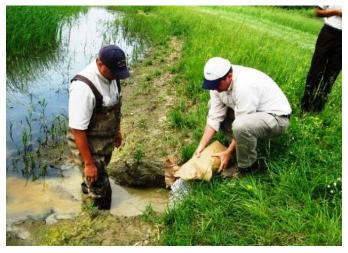
Photo 5. Manual addition of AquaBlok from a 50lb bag.
