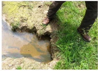
Photo 2. A top-down perspective of the breach in the earthen berm separating an inundated wetland (left) from an adjacent non-inundated wet prairie environment at drawdown (right).
