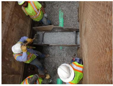
Photo 1. AquaBlok placed into the trench dam form, and being leveled off on top prior to adding fill aggregate on both sides of the form.
