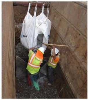
Photo 5. AquaBlok placement from a bulk bag – note the bag was cut open from the side as the full bag was not going to be used at once and the contractor did not feel they could close off the bottom spout safely once opened.
