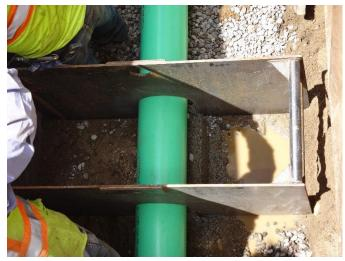
Photo 3. Positioning of the trench dam form prior to adding AquaBlok material.
