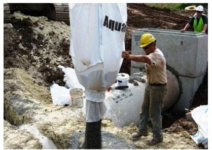
Photo 1. AquaBlok placement from a bulk bag (standard shipping unit for bulk material) using a track loader/excavator – note discharge snout directing product into trench cut perpendicular to the overflow discharge pipe
