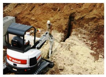
Photo 3. Positioning of the AquaBlok above the anti-seep trench (basin to the right)
