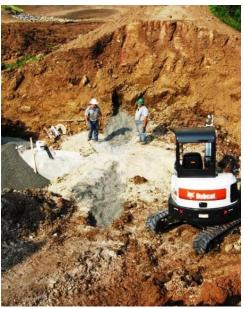
Photo 5. AquaBlok filled anti-seep trench from atop existing berm (lift one of three, ~6 vertical feet of the ~18 vertical feet total
