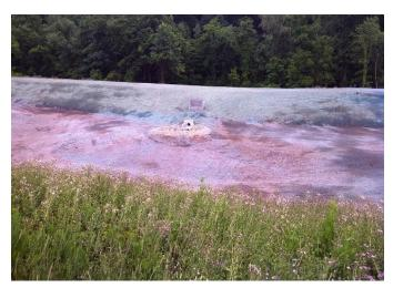
Photo 7. Berm reconstruction completed (basin in foreground) - note riser structure in center of photo
