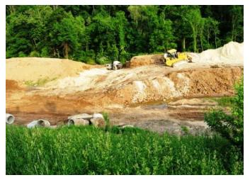
Photo 6. Berm reconstruction in process (basin in foreground)
