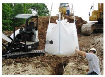
Photo 2. Excavation of the perpendicular anti-seep trench (~12" width) that ultimately received AquaBlok from atop the existing berm (basin to the left)
